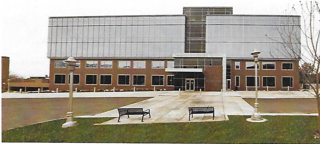
Warnock Engineering Building
