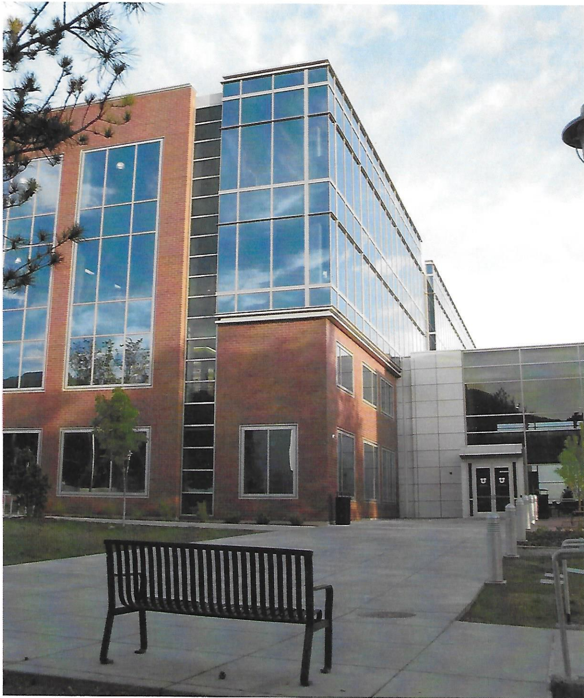
Warnock Engineering Building
